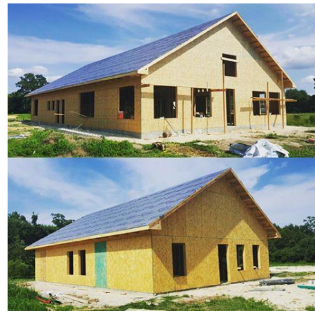
The current state of The Anchor House
